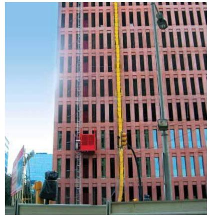
Used with the purpose of carrying material and personnel to filoors with its completely closed cabin.
