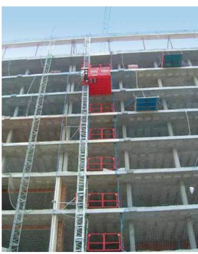
Encomat IZA 1500 is a material hoist designed in such a way that it can enable ease in your construction works with its quicker and more secure system when compared to hoists with rope system. Operates with high and secure performance on its rock and pinion mechanism. By adjusting its floor-stop mechanism from electric panel you can allow it to stop in the intended floor. Model with the wide cabin provides ease in carrying plaque and panels.
